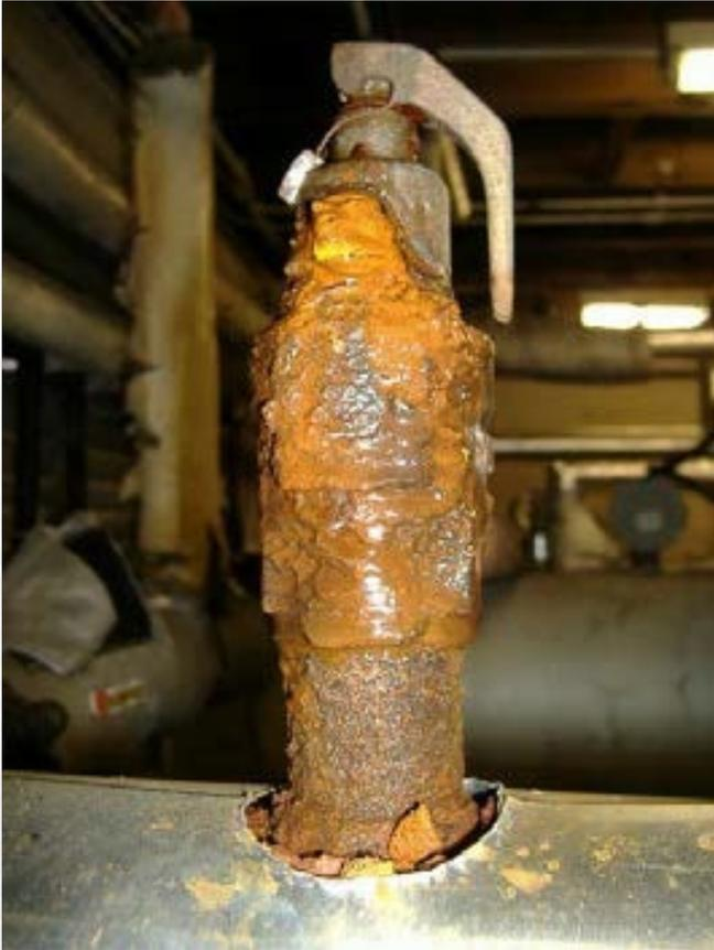
Corrosion caused by damaged diaphragm
