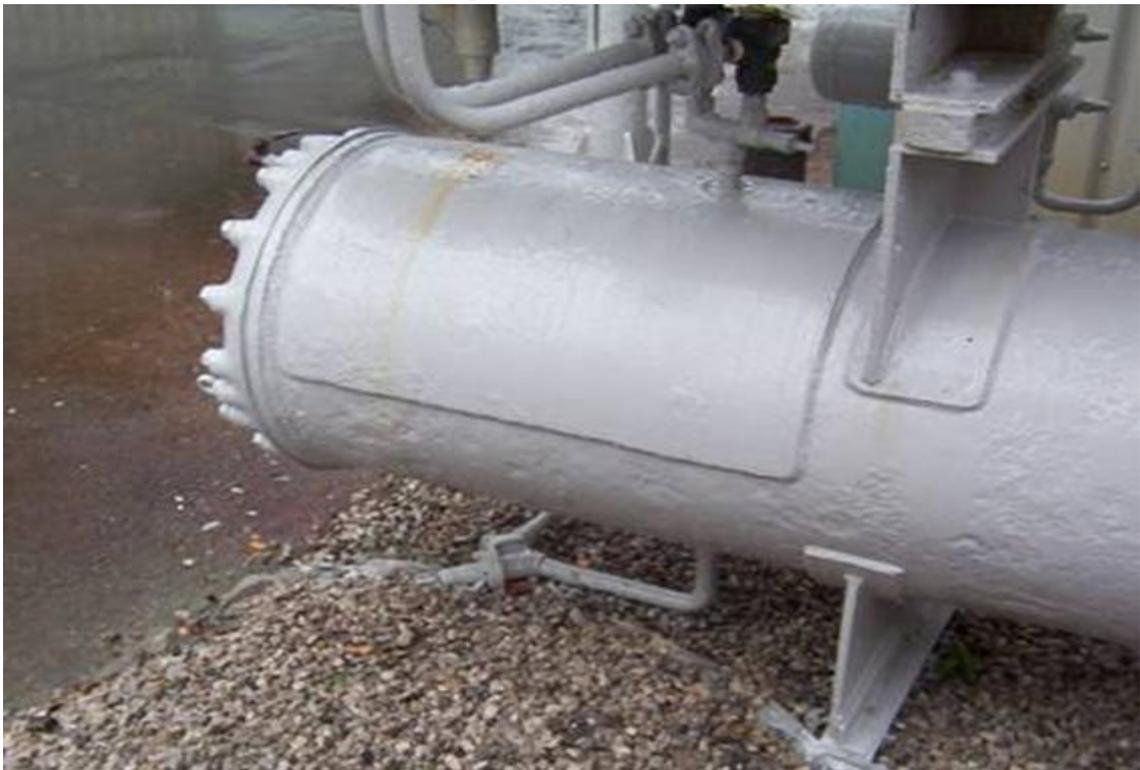
**Use of a fillet welded temporary repair over corroded region of heat exchanger**
