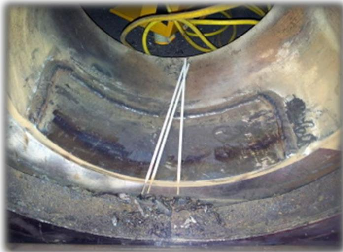
The preferred type of repair for a fatigue crack (either at toe of a fillet weld or root of a single-sided weld) at the corner joints on shell boilers is to use a ‘D’ patch. For cracking into the tube plate it will generally be necessary to remove a ‘D’ patch from the furnace to gain access to the crack for a grind and weld repair.
