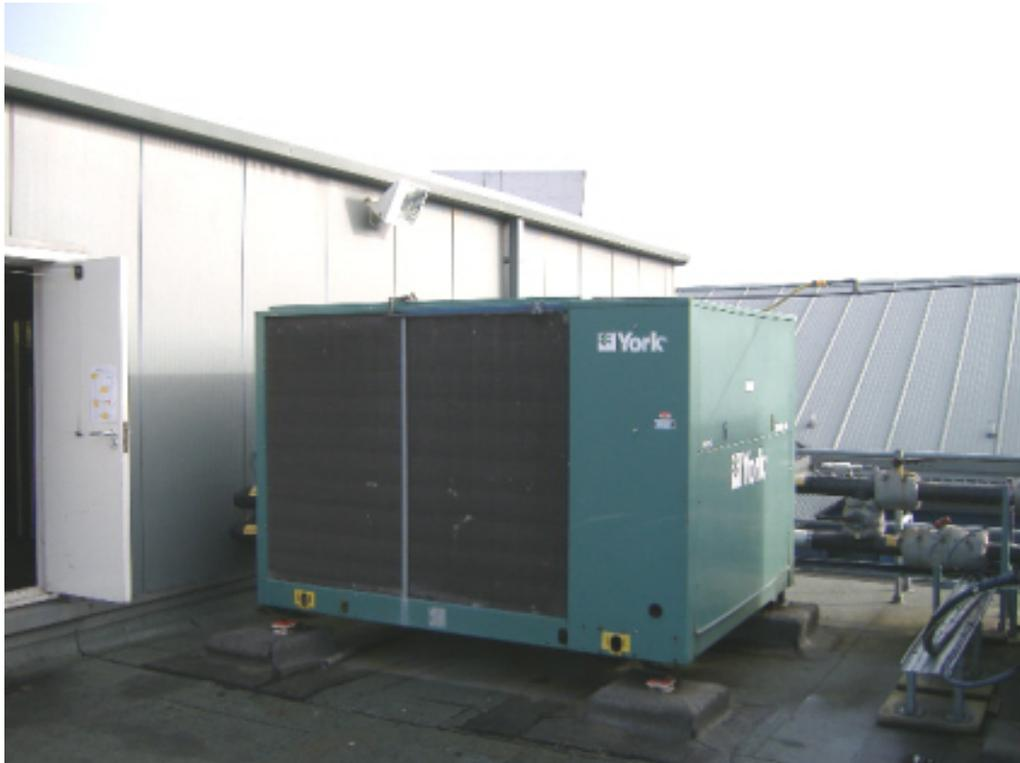
**Picture 1 — Typical packaged refrigeration system**
