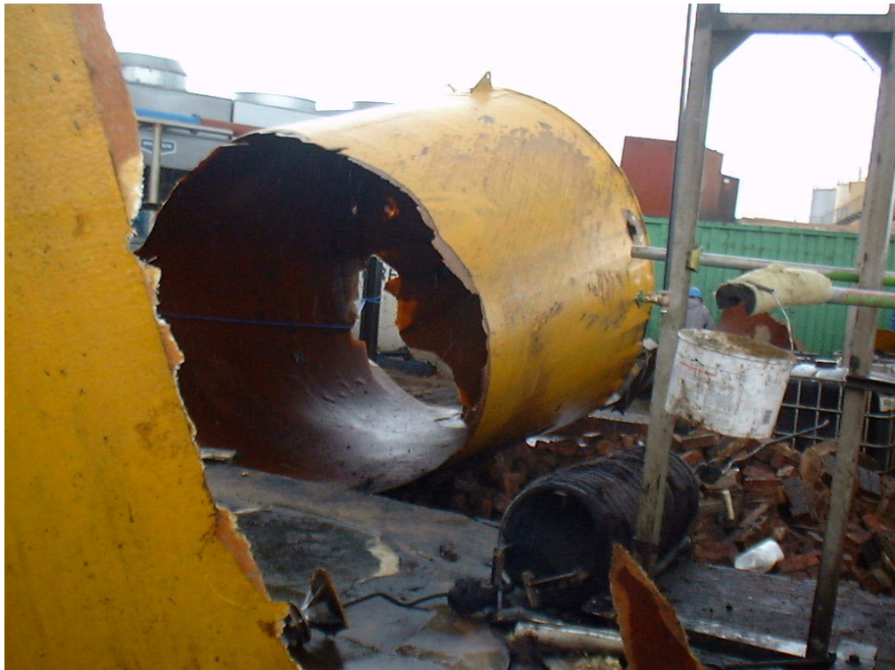
Picture 6 - Historical image of a catastrophic failure
