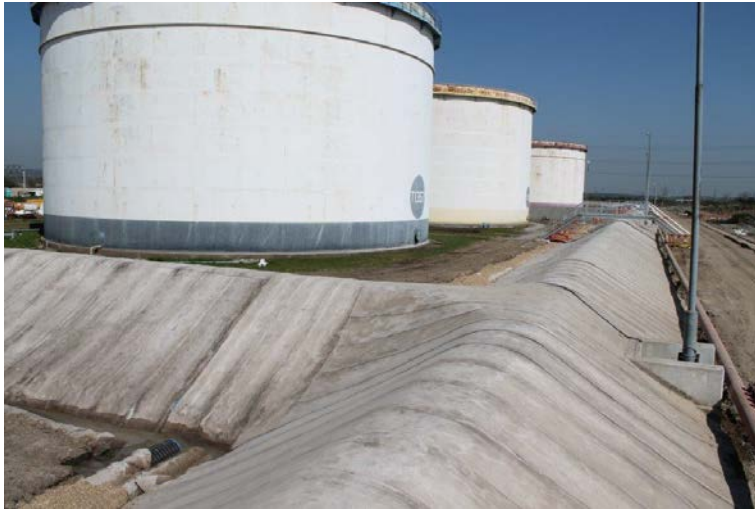
Example of earth / concrete mound
