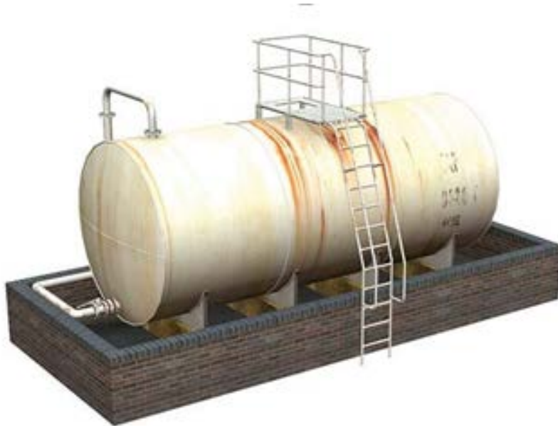
Example of walled bund
