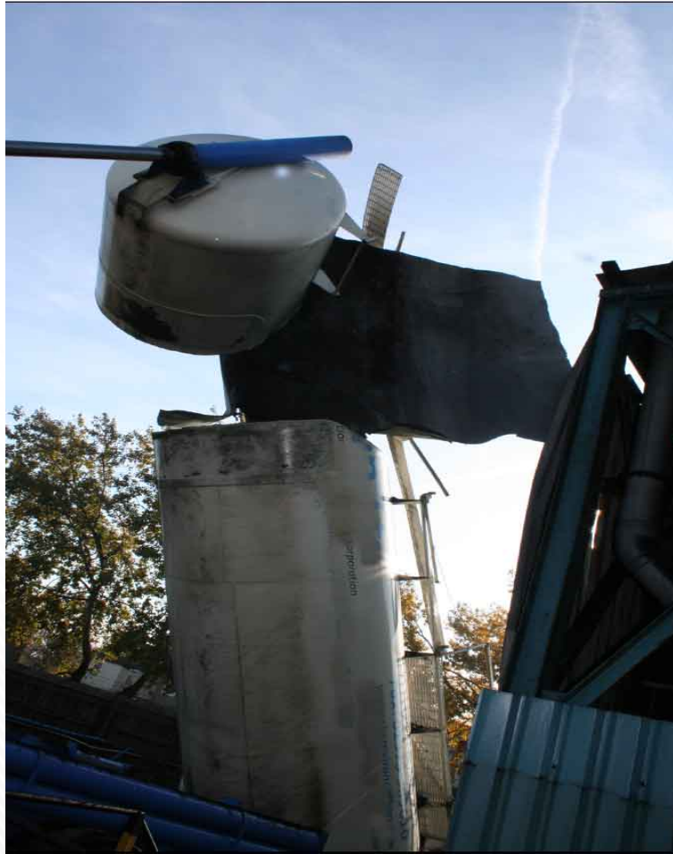
Failed tanker in the upright tipping discharge position
