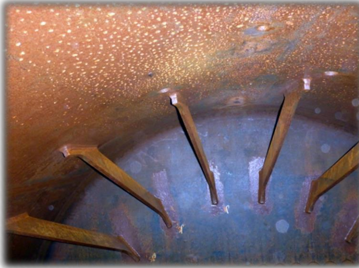
Typical image of gusset stays
