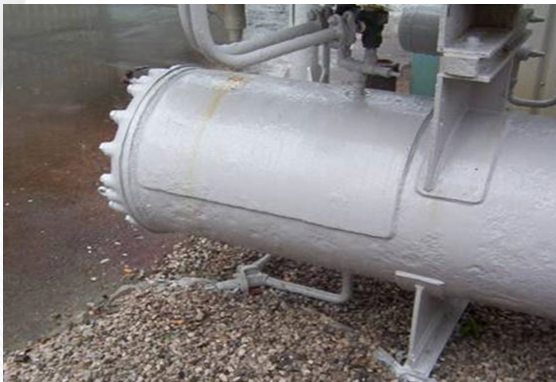
Use of a fillet welded temporary repair over corroded region of heat exchanger
