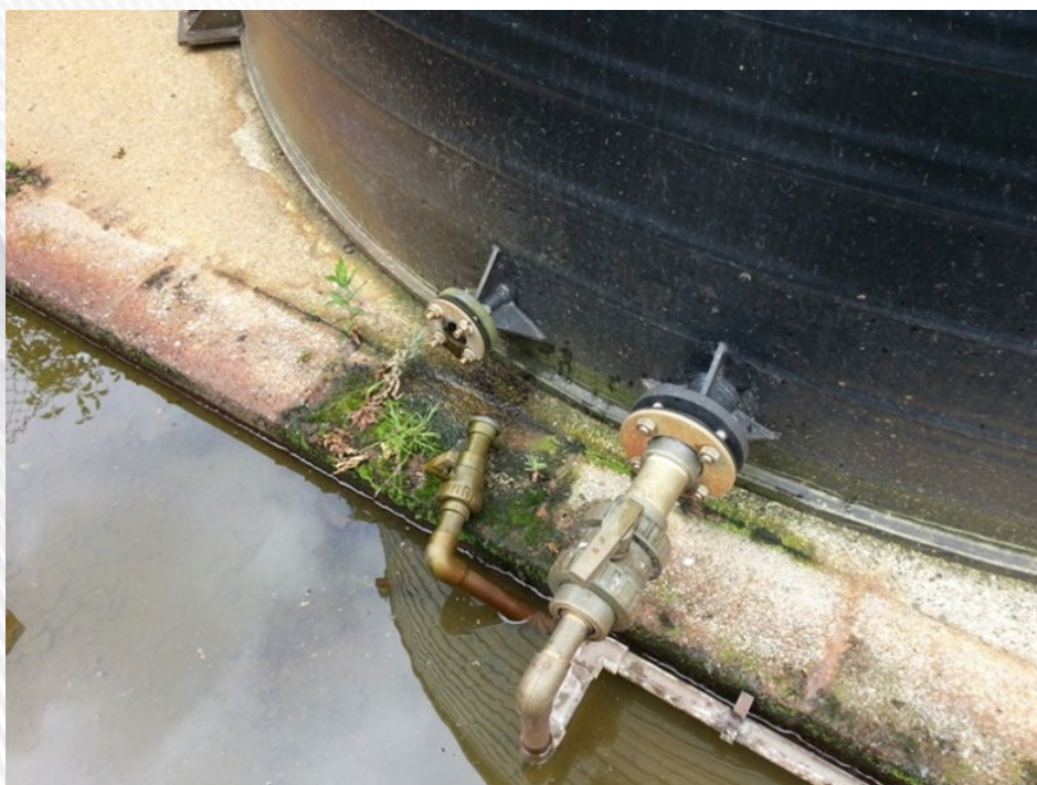
Picture 7 - Fatigue crack induced by manufacturing defect, which has propagated
