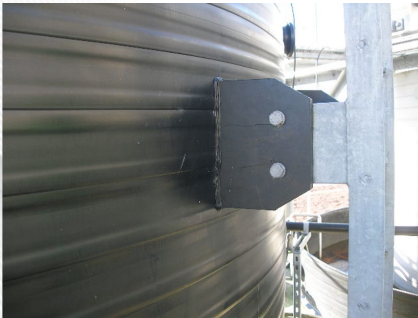
Picture 1- UV degradation – note the change of colour
