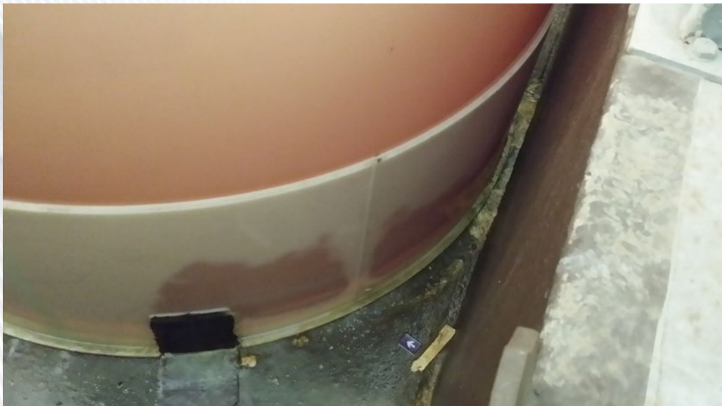
Picture 4 - Discolouration due to polymer or molecular degradation
