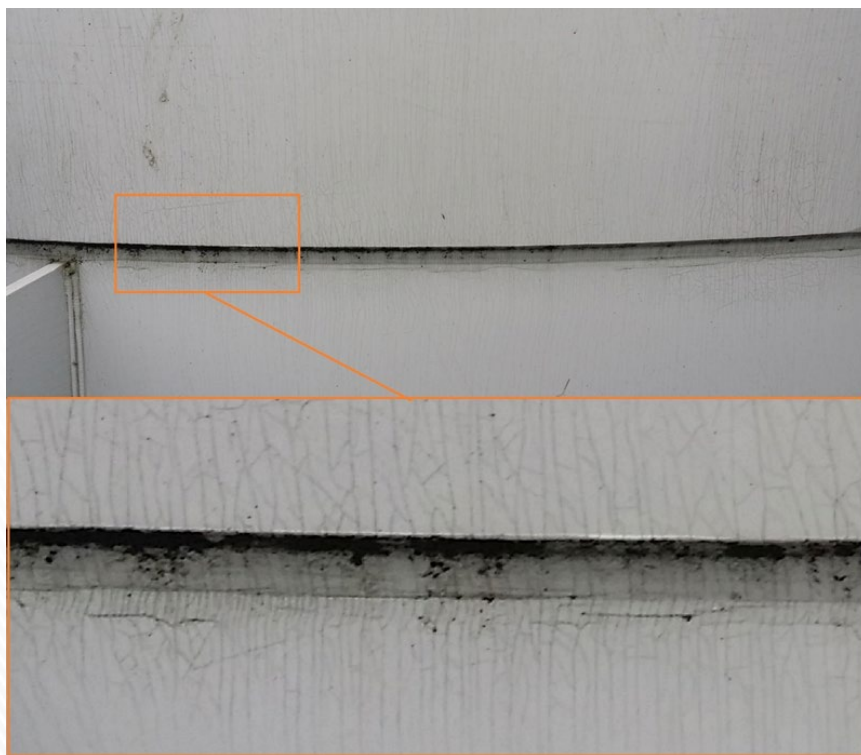
Picture 5 - Degradation due to UV – note the multiple fine cracks
