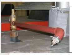
The discharge pipe is plugged! Why? Because when the valve lifts it unscrews itself from the equipment! (Due to the reaction force and no restraint on the pipework)
